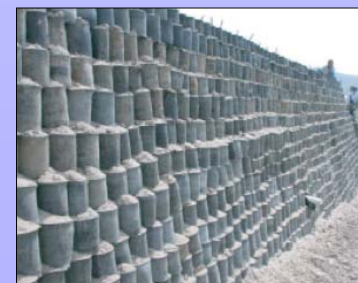
Wall made of recycled tires in Tijuana, Mexico
