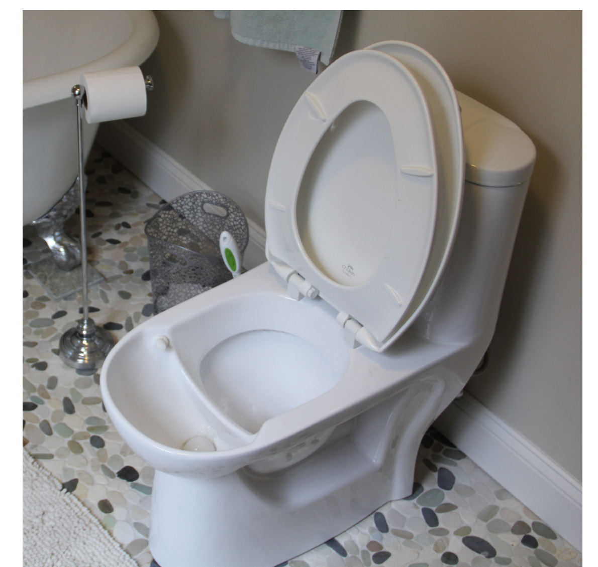
Urine diverting toilets have a divider built into the bowl so that urine can be captured separately in a special storage container and later removed from the watershed. Around 80% of the nitrogen from human waste is excreted in urine.
