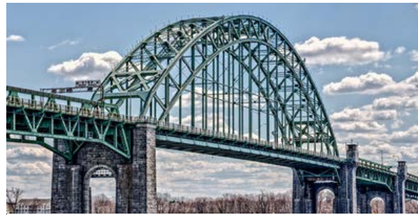
Figure 1: Steel Tied-Arch Bridge
