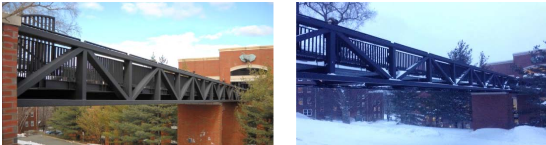
Fig. 1 South view of Dowling Hall Footbridge
