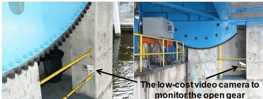
Figure 2. The open gear of the movable bridge and the video camera for lubrication monitoring
