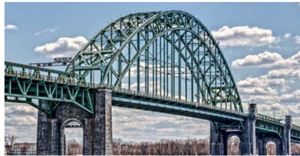
Figure 1: Steel Tied-Arch Bridge
