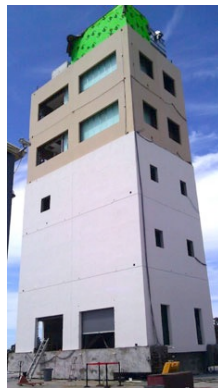
Figure 1. BNCS building on University of California San Diego’s outdoor shake table.
