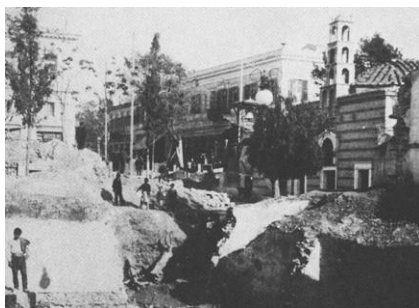
Figure 20. 1895, Pantanassa, during the construction of Monastiraki station of the Electrical Railway
