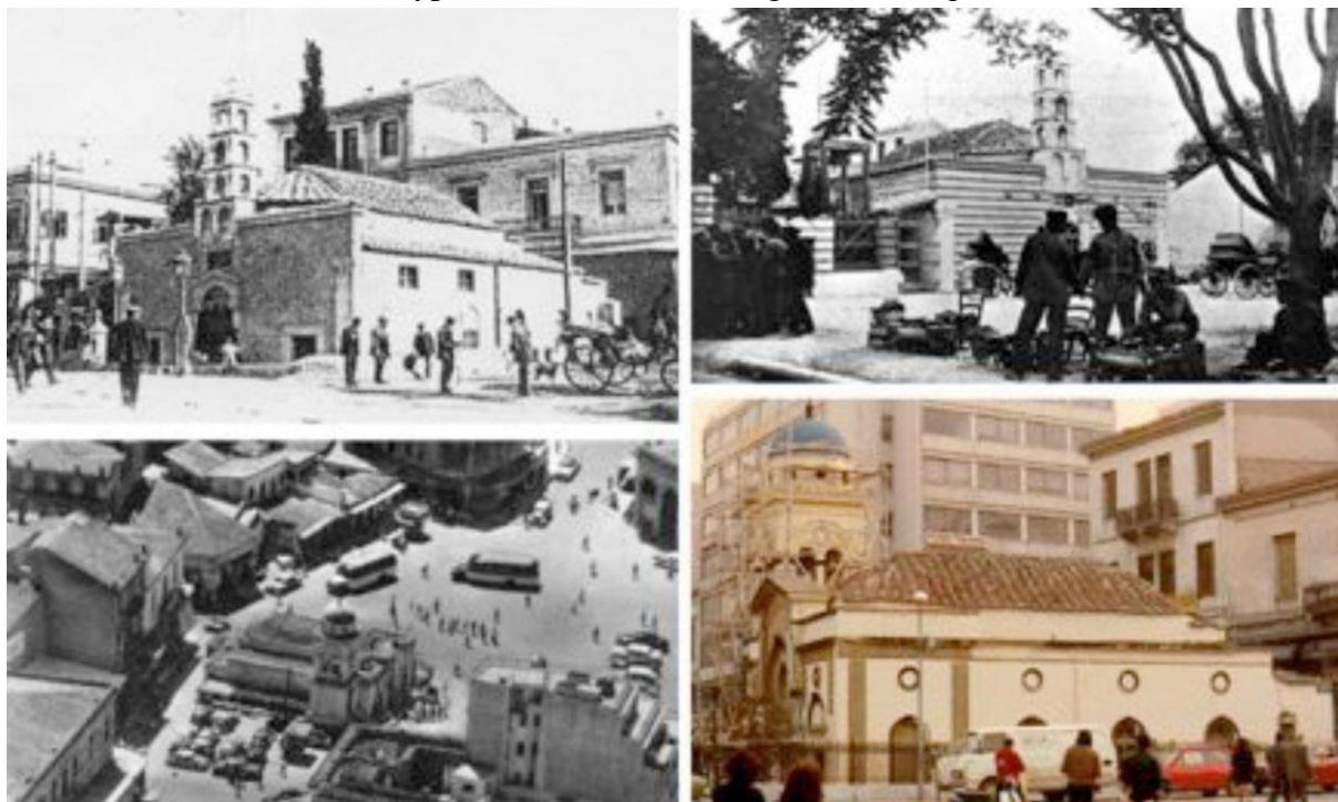
Fig.22. Successive transformations of Monastiraki square. Down on the left the left 1958, Down on the right 1983.
