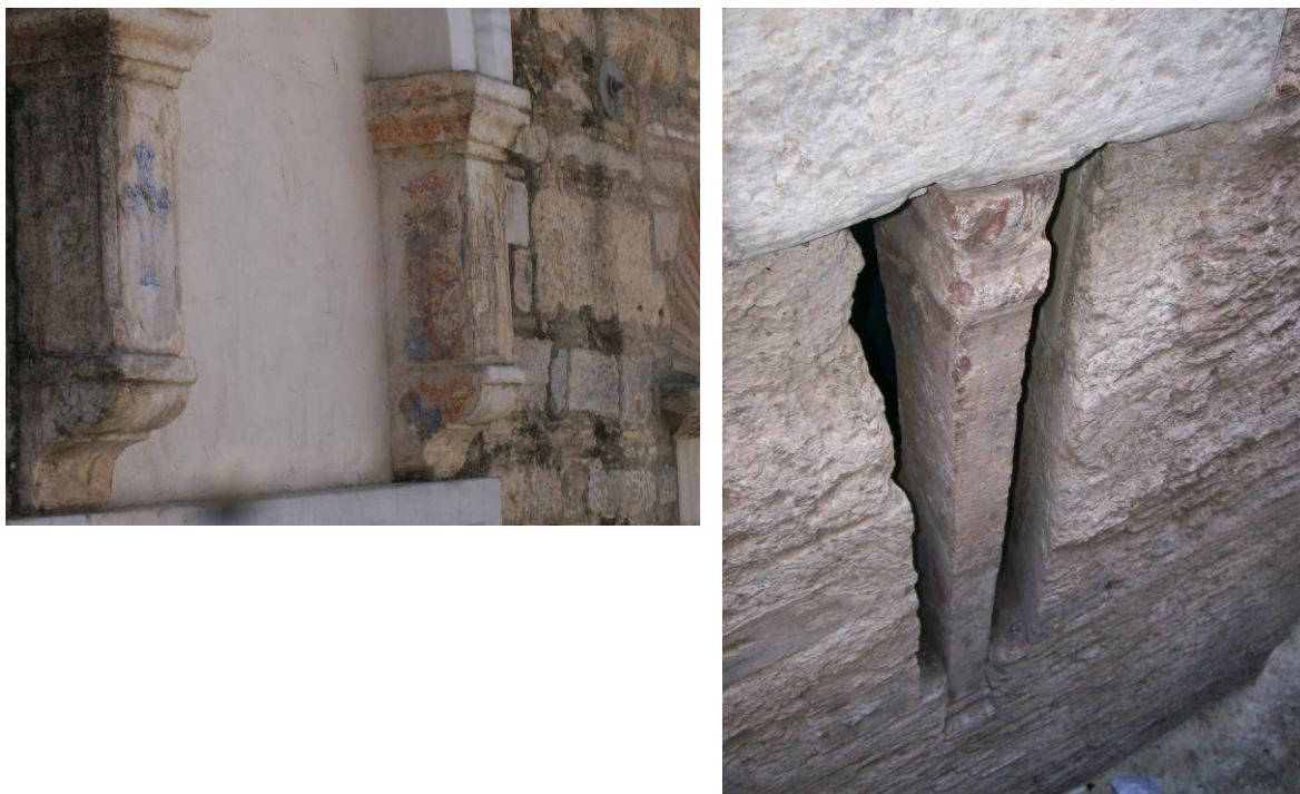
Fig.29. In 1911, during some restoration works they have moved from the church some spolia in marble, from their position in origin. Then they rebuilt them at other positions (Photos taken from N.DELINIKOLAS, Restoration of the church of Madonna Pantanassa, contrast of principles)
