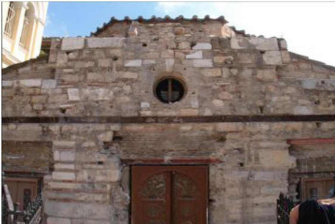
Fig.28. Main western façade during 2004-2006 restoration works (Greek Ministry of Culture)
