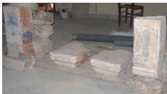
Fig.25. Rebuilding the main entrance (Photos taken from N.DELINIKOLAS, Restoration of the church of Madonna Pantanassa, contrast of principles)
